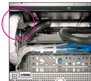
Cinch Tie mounted within cabinet UGTC3S-X10
